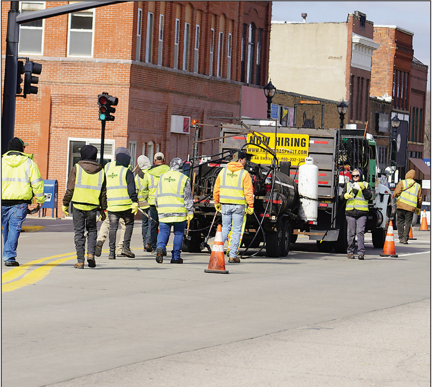
Iowa DOT workers patched up Highway 9/Central Avenue at the end of April into the beginning of May
