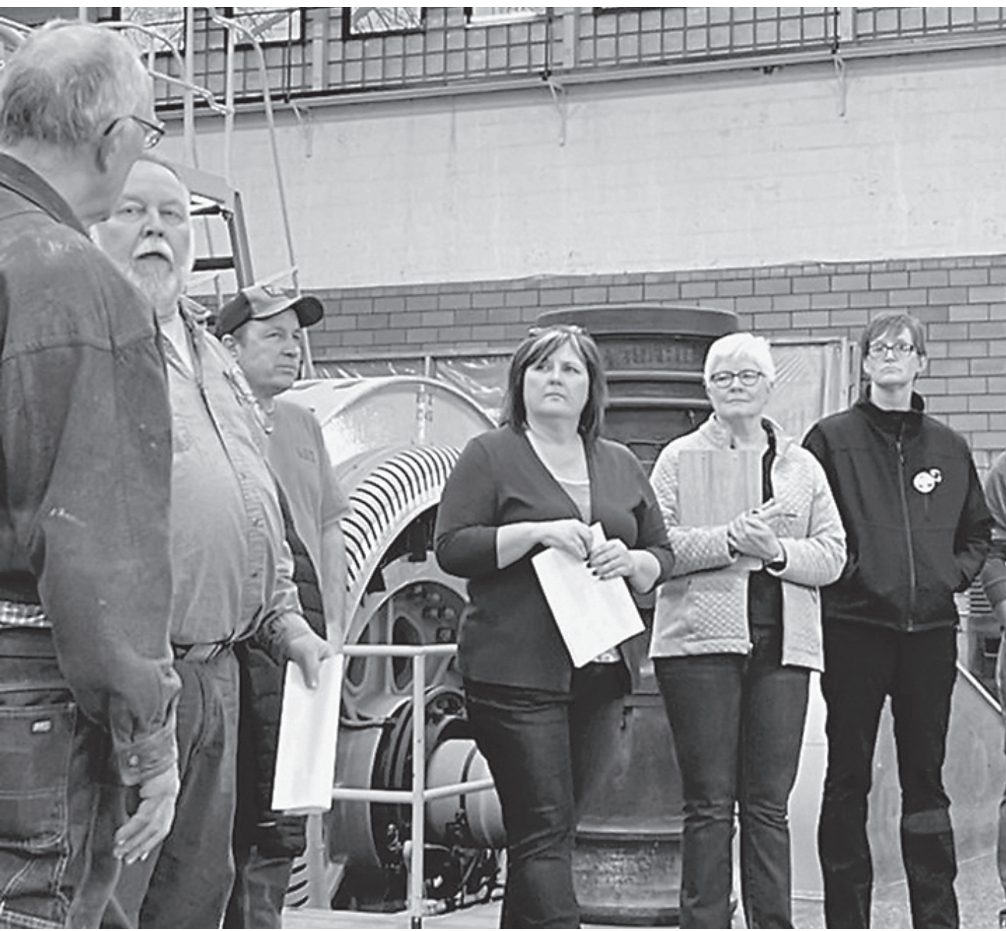
Bret Mace, electric foreman, second from left, talks to council member Roy Gage about the electrical production plant. Dale Bradley, electric operator/mechanic, Penny Clayton, city administrator, Beth Burton, city clerk, and council member Joan Heckard were also on the tour.
