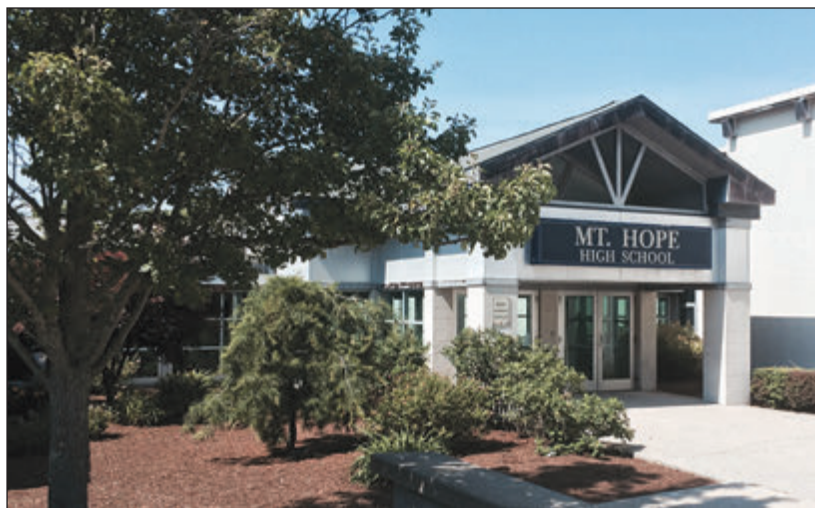
A failed sprinkler pump caused extensive water damage at Mt. Hope High School.
