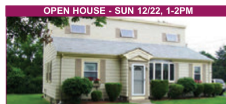
(90 Bellview Ave) Tiverton - Beautifully maintained Cape with open floor plan, hardwoods, 1st floor bedroom. Large expanded second floor includes in-law set up. Well landscaped yard, large mahogany deck, shed and oversized garage. $299,000
