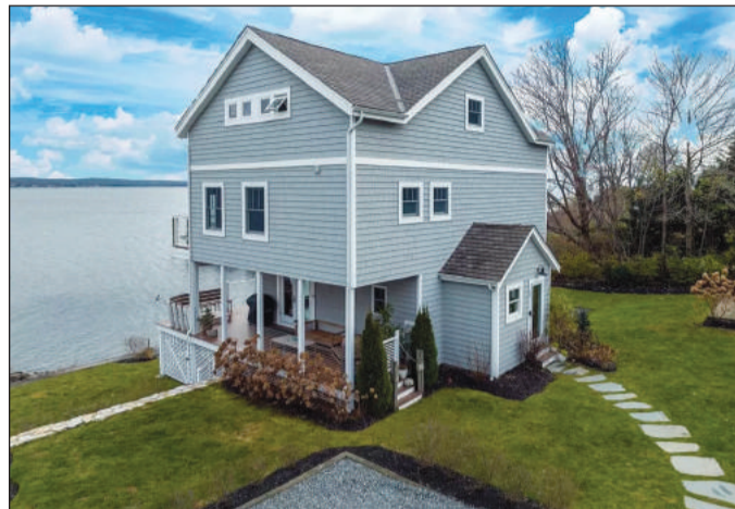
This custom home overlooks the Sakonnet River in Portsmouth, with water views from every room.
