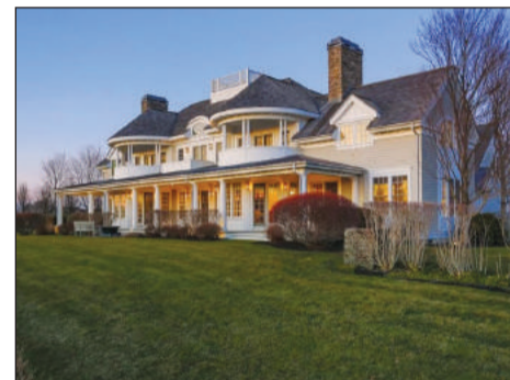
The rear of the large property includes patio, enormous deck and multiple balconies off of the second-floor bedrooms.
