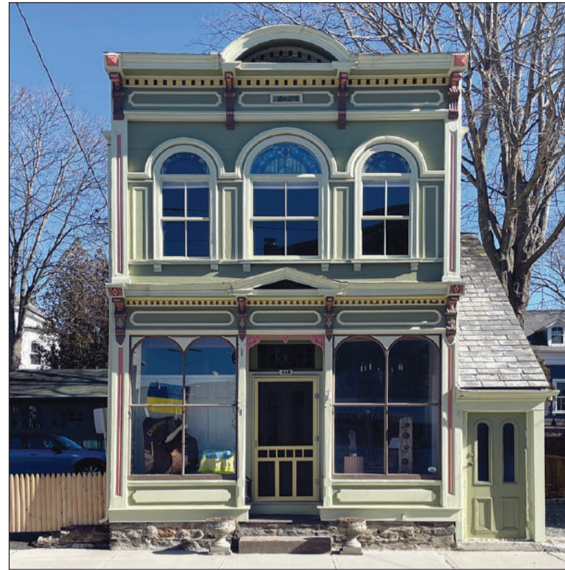
Dickey photographed 146 Water Street and dedicated an entire post to it, writing, "This little commercial building is likely the best preserved little shop in all of Rhode Island. What really makes it special is that it sits on a street with several other, small-scale and well preserved commercial buildings. Together, they provide a sense of what it was like to live in 19th-century coastal New England."
