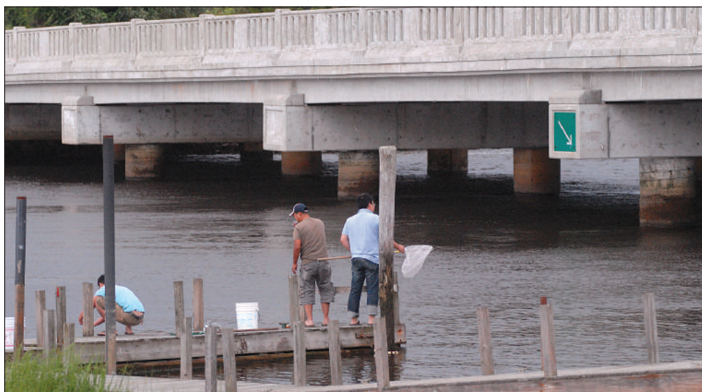
A long awaited feasibility study on the need to dredge around Hix Bridge is nearly complete, selectmen were told at a meeting last month.
