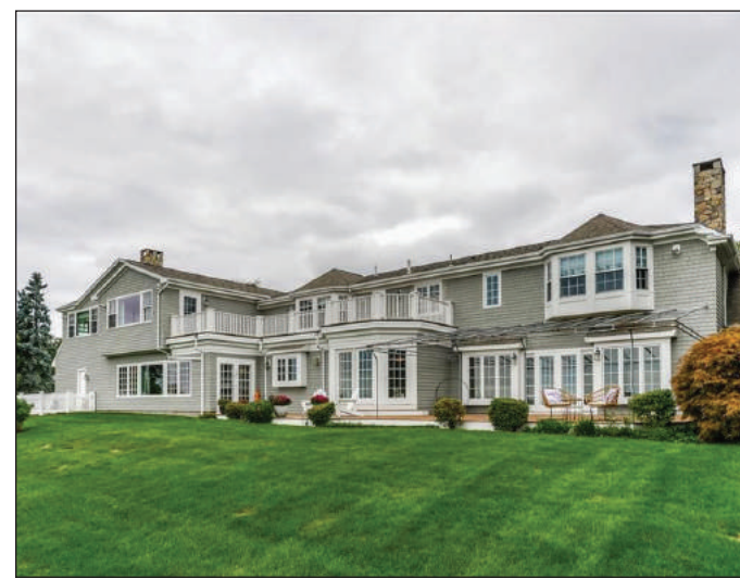
The rear of the house features decks on both levels, all facing south to Narragansett Bay.
