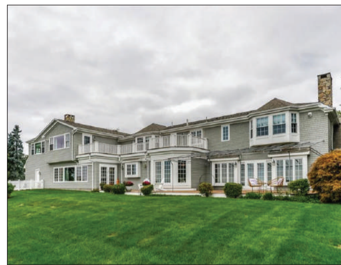
The rear of the house features decks on both levels, all facing south to Narragansett Bay.
