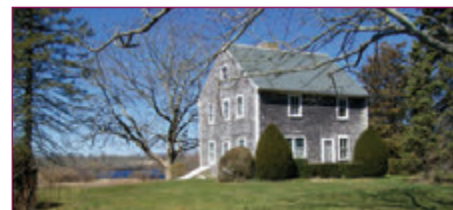
South Tiverton - Near Little Compton line - 9 acre farm overlooking Nonquit Pond. Antique home in need of restoration, barns, garage, and beautiful yard with stone walls. $1,199,000
