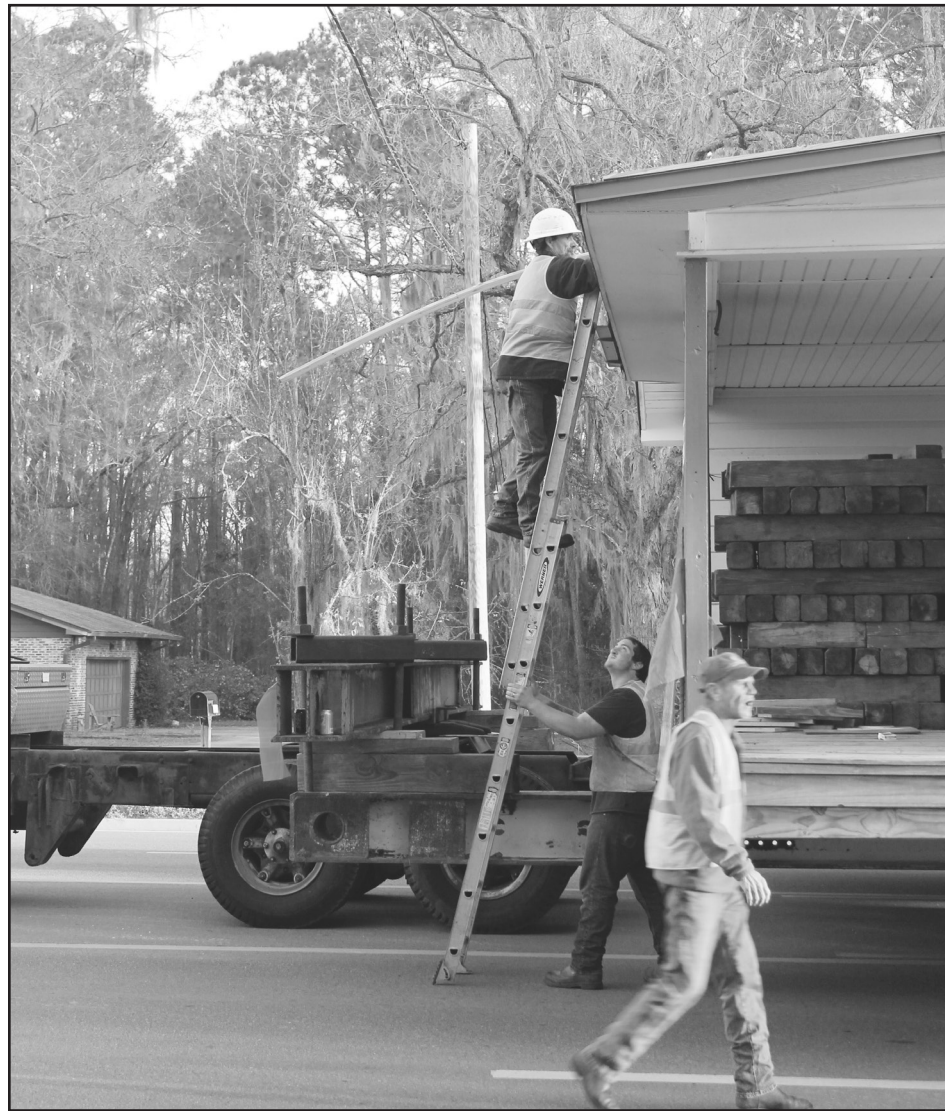
A work crew member for Hygema House Movers places a special wooden board atop the home to allow safe passage under any power lines en route to its new site on Bronco Road in Middleburg.
