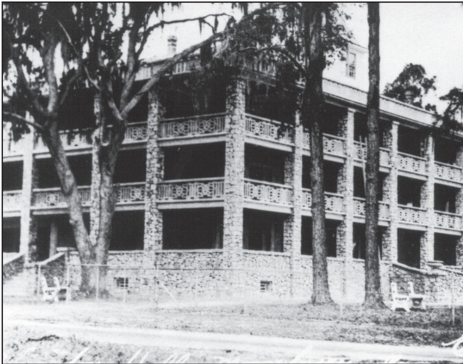
After construction of concrete porches and a coat of pearl dash stucco the former Victorian styled, clapboard Hotel Marion at the southwest corner of River Rd. and Kingsley Ave. became Moosehaven's Brandon Hall.
