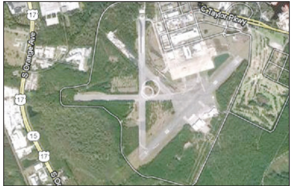
This aerial shot of Reynolds Industrial Park shows the landing strip that could be transformed into a new county airport if 2017 plans to do so are not scrapped.
