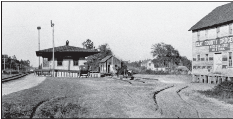
In 1932, the most recent Masonic Lodge in Clay County was chartered in Orange Park. Meetings were held in the second floor of the Farmers' Co-operative building, which still stands at the northeast corner of Kingsley and Railroad Avenues. Originally, the train station was conveniently next door.
