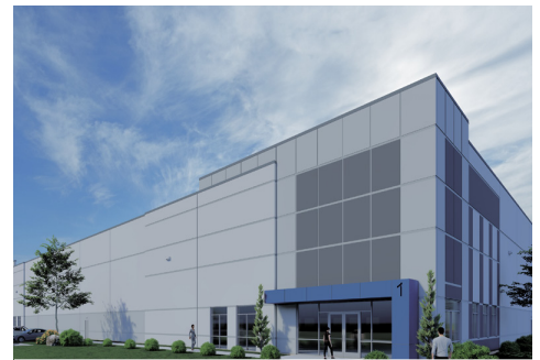
First Gulf | Jacksonville, FL 109,200 SF Speculative Warehouse
