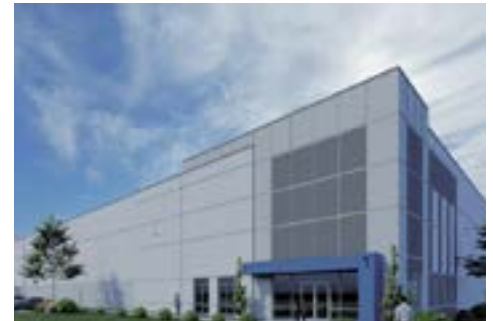
First Gulf | Jacksonville, FL 109,200 SF Speculative Warehouse
