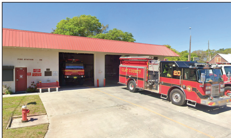
How the current Fire Station 20 looks like.
