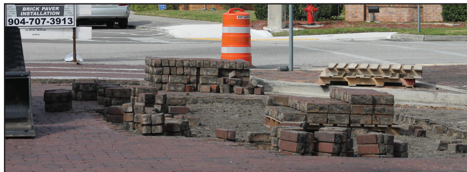
Some of the improvements planned include widening sidewalks to fifteen feet.
