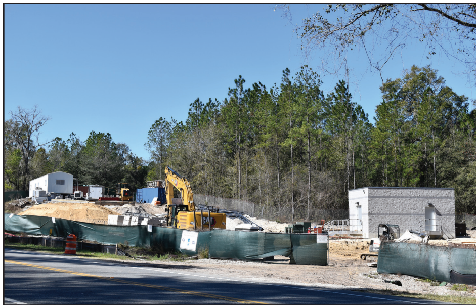
Work on the pump station for the Black Creek Restoration Project is moving along without any major setbacks. At the current pace, water should start flowing from the South Fork of the Black Creek into lakes Brooklyn and Geneva this time next year.
