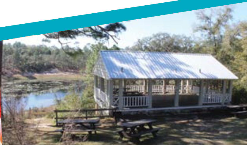
Park Pavilion at Gold Head State Park
