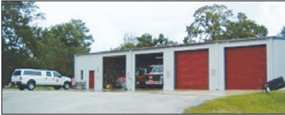
Lake Asbury Fire Station
