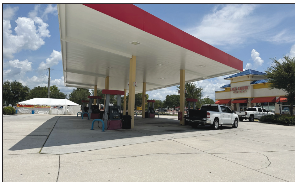
The Lake Asbury Food Mart usually is busy with customers getting quick treats and gasoline, but the store said one day it averaged less than two customers an hour because of the work being done to widen Sandridge Road.
