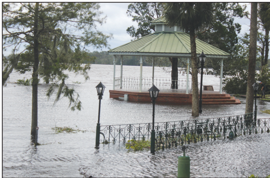
Hurricane Irma led to some flooding and erosion in Green Cove Springs in 2017, especially here at Spring Park. Hurricane season runs through the end of November.
