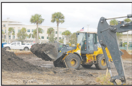
Crews started the project more than two years ago.
