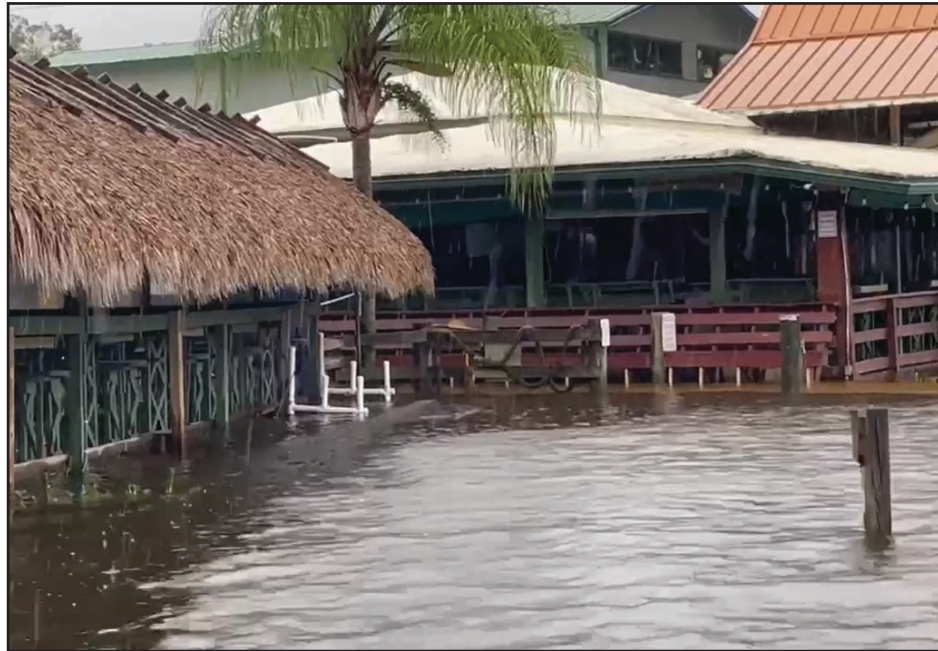
Minor flooding was reported at Whitey's Fish Camp on Fleming Island.
