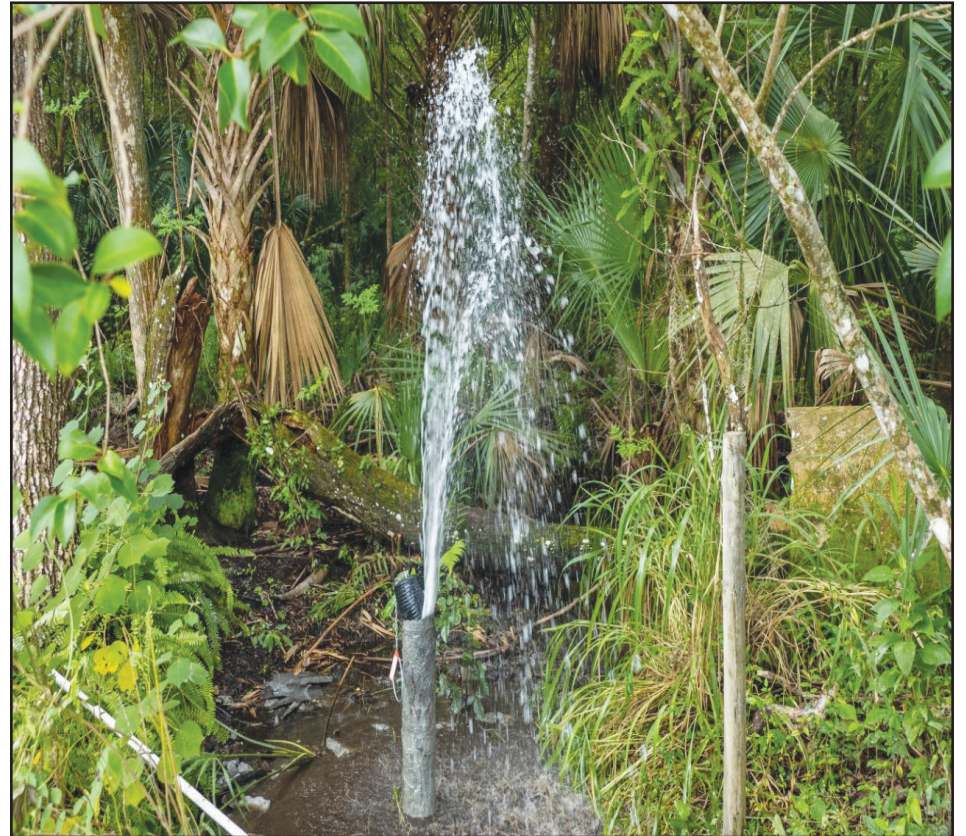
The St. Johns Water Management District agreed to stop assessing fees to cap abandoned free-flowing artesian wells to permanently stop the waste of water. So far, more than 3,000 wells have been capped, saving the district more than 745 million gallons of water.
