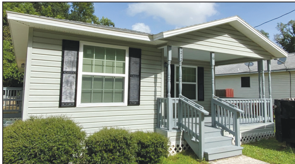
After sharing one bathroom with seven people at her parents' house for years, this house on Houston Street was remodeled to provide the first home for a mother and her 3-year-old son. The project was made possible by Habitat for Humanity and hundreds of volunteer hours.
