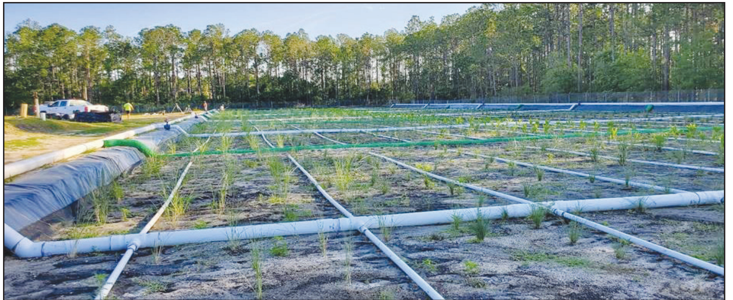
A system of tubing at the Doctors Lake Phosphorus Removal Pilot Project is operational and working to reduce the levels of dissolved phosphorus by 90% to help lessen the threat of algae blooms in the inlet.
