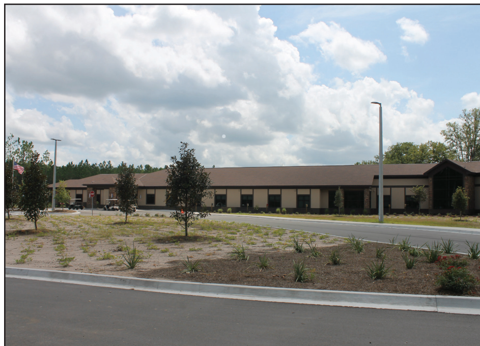
The new Pavilion at Penney Farms has 50 beds and 24-hour nursing care. The $10 million building opened two weeks ago.
