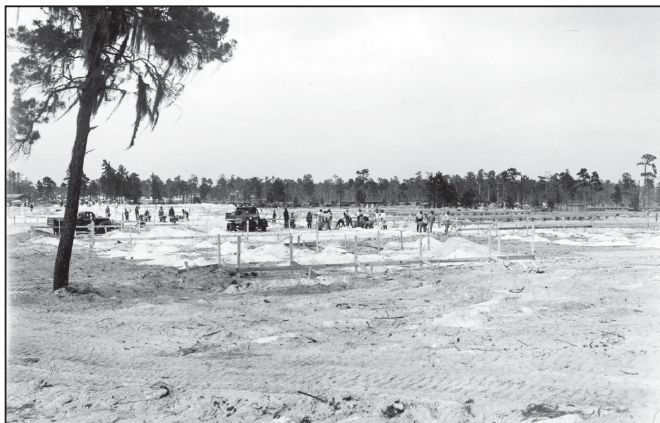
Workers lay the early groundwork for Camp Blanding. When soldiers were training at the massive complex, it was considered the fourth largest city in Florida.
