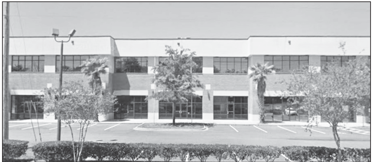
Plans are nearly completed for the new Veteran's Association Clinic in Middleburg. Construction is scheduled to start in a couple months for a facility for the 30,000 veterans in Clay County. Mental health, primary care, lab draws are among the services that will be included. Voting to name the clinic can be done at the Clay County Supervisor of Elections Office or by calling Rep. Ted Yoho's office at (352) 505-0838.
