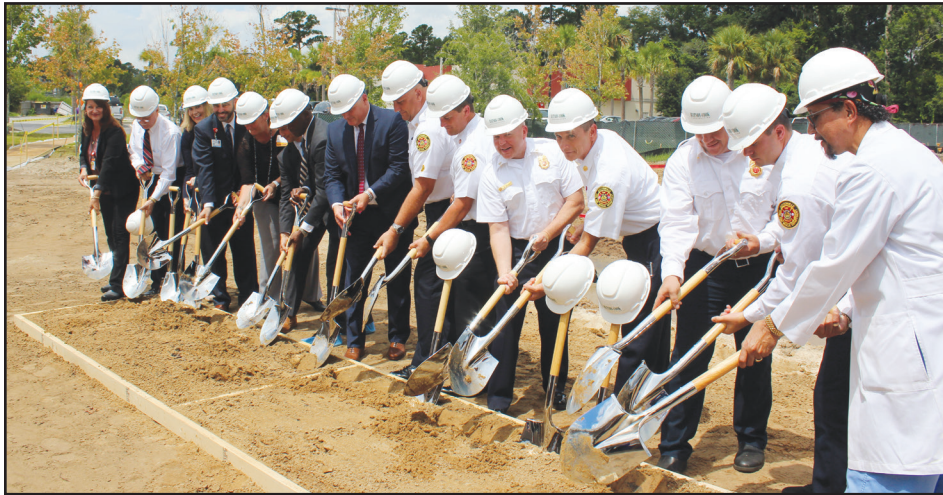
OPMC's newest stand-alone ER should be complete by the end of 2018. The $12 million facility will have 10 beds and employ about 50 staff.
