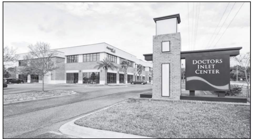
One of three buildings at 400 College Dr. in the Doctors Lake Center will become home to a new VA Clinic, a project announced Aug. 1 by U.S. Rep. Ted Yoho(R-3), who has been working on this for three years.
