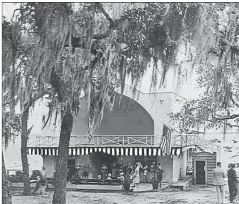
This is a photo from 1925 when the Keystone Beach Pavilion was in its heyday complete with bandshell. The Heritage Commission is gearing up to commission a study to determine the feasibility – including costs – for restoring the treasured structure.
