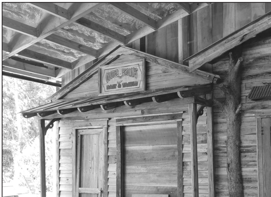
Construction continues on the back patio of Boondocks Grill and Bar. Owners are planning to open next month.
